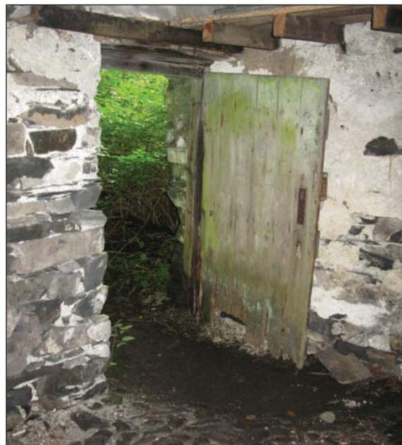
The front door. Falling apart and off its hinges
